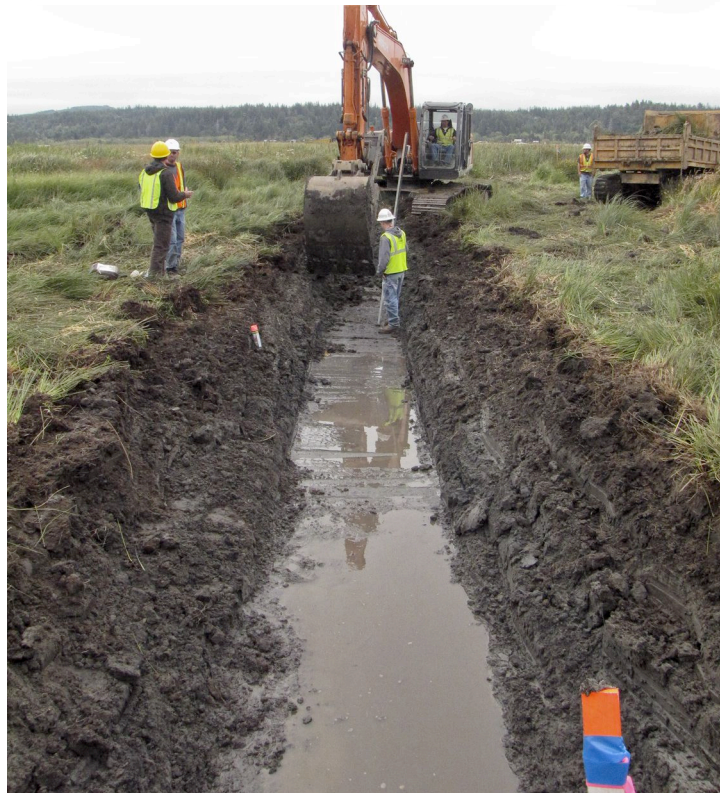
Channel Excavation. Photo by R.W. Lowe
