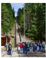
Greetings and introductions accomplished we embarked on a short hike to a location near headquarters where an early innovation in hands-on study was impressively on display. Constructed in 1991, the debris-flow flume allows for the artificial creation
