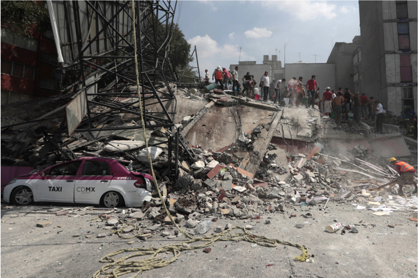
Volunteers search a building that collapsed after an earthquake in the Roma neighborhood of Mexico City on 19 September 2017. Photo by Eduardo Verdugo/ AP
