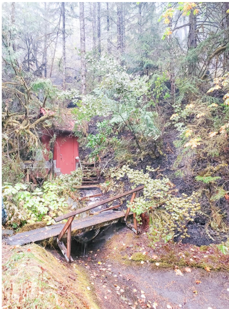
Gage station at HJ Andrews Experimental Forest. The Holiday Farm Fire almost reached it.
